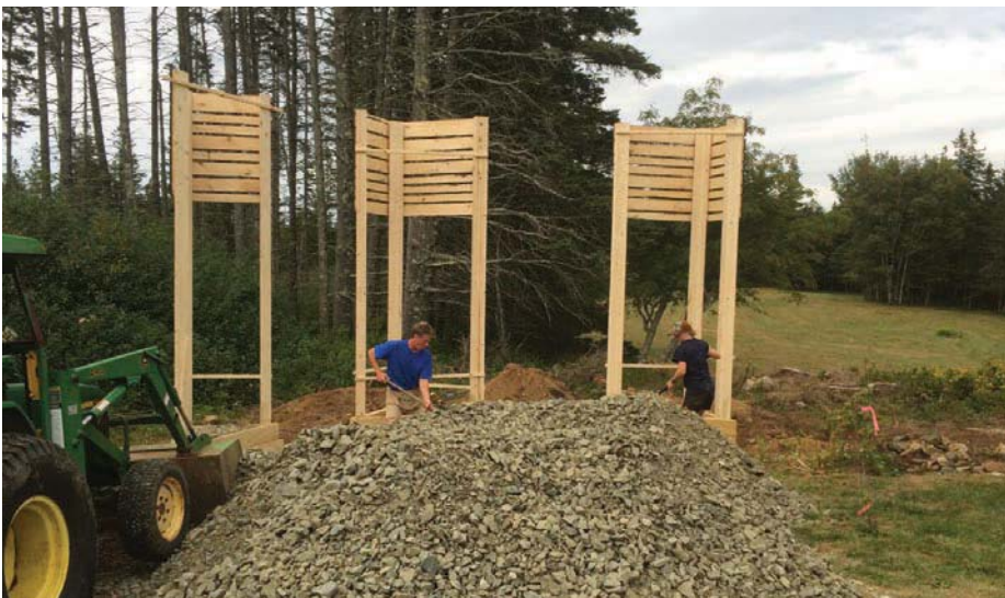
••••••■ Day 8: Assembly on site at North Haven Community School
